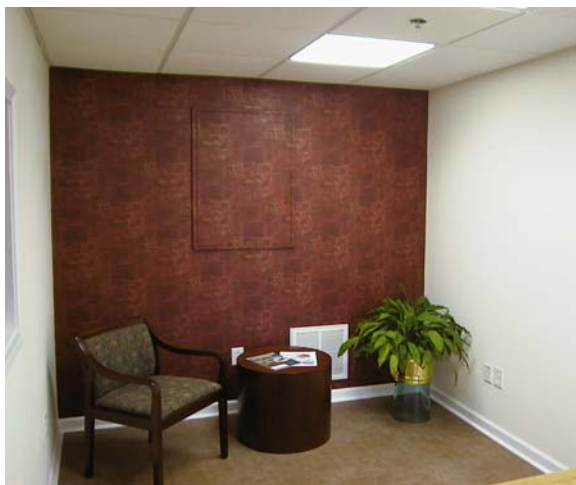
Wall Covering Applied To Access Panel
