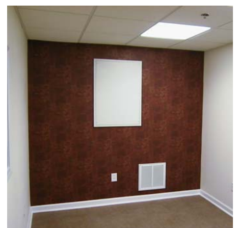
Decorative Access Panel Installed
