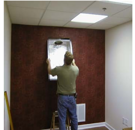
Installation of Sleeve
