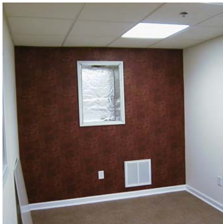
Sleeve Installation Complete
