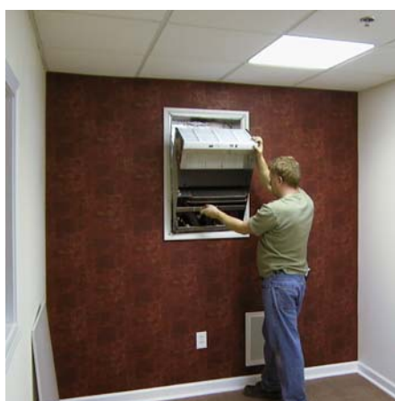
Refrigeration Chassis Installed
