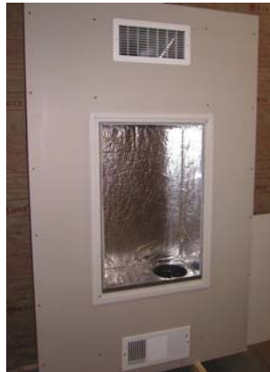
5. Finished Drywall with Frame & Grills
