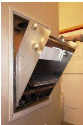
7. Installing chassis into sleeve
